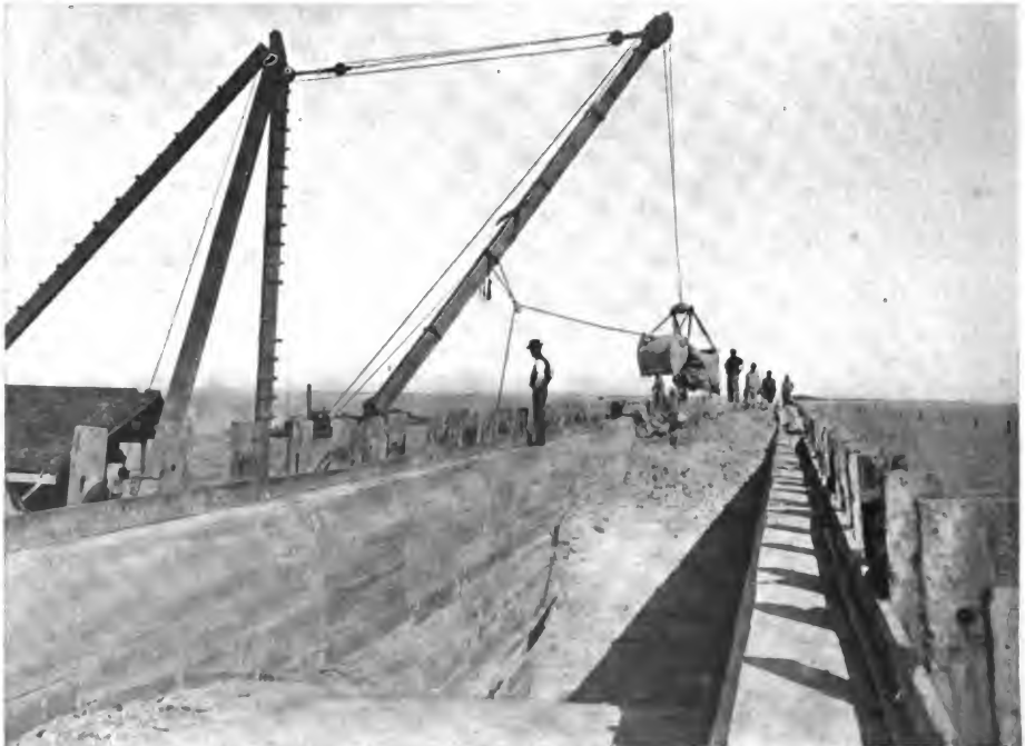
Long Key Viaduct.—Filling the last arch.
